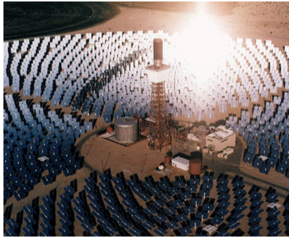
Concentrated Solar Power
